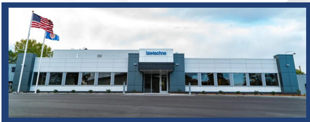
Bio-Techne 55,000 sq. ft. animal-free GMP facility located in St. Paul, MN USA
